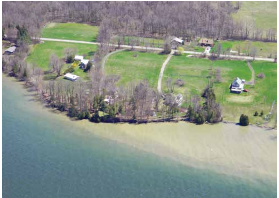
Figure 4. Shoreline erosion along the west shore of North Hero, Vermont, during record-breaking flooding in 2011 on Lake Champlain. Photo: LCBP.
