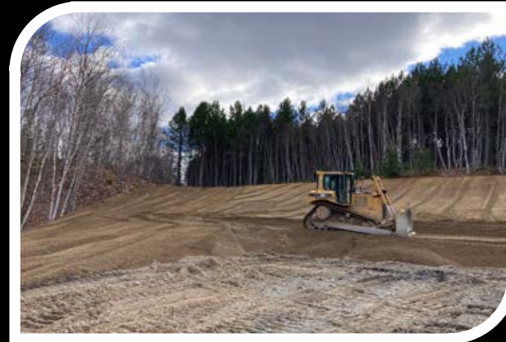
Slopes stabilization (October 2022)
