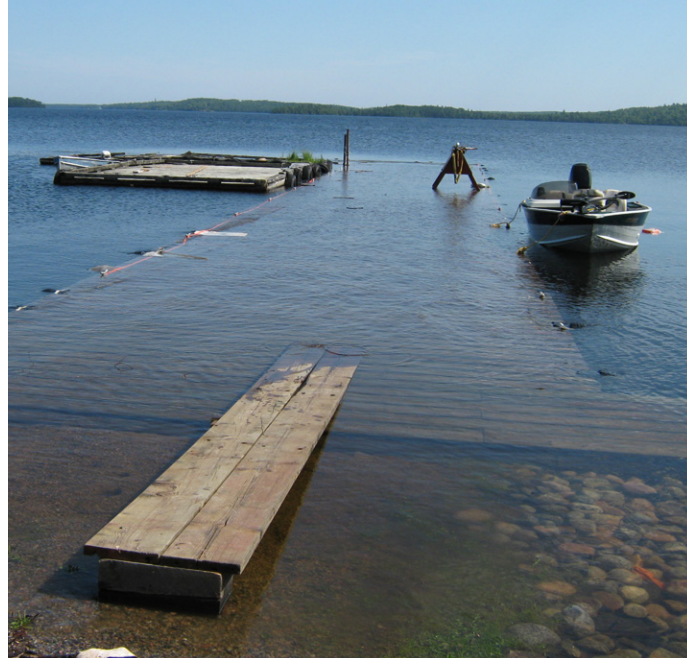
High water dock impacts
