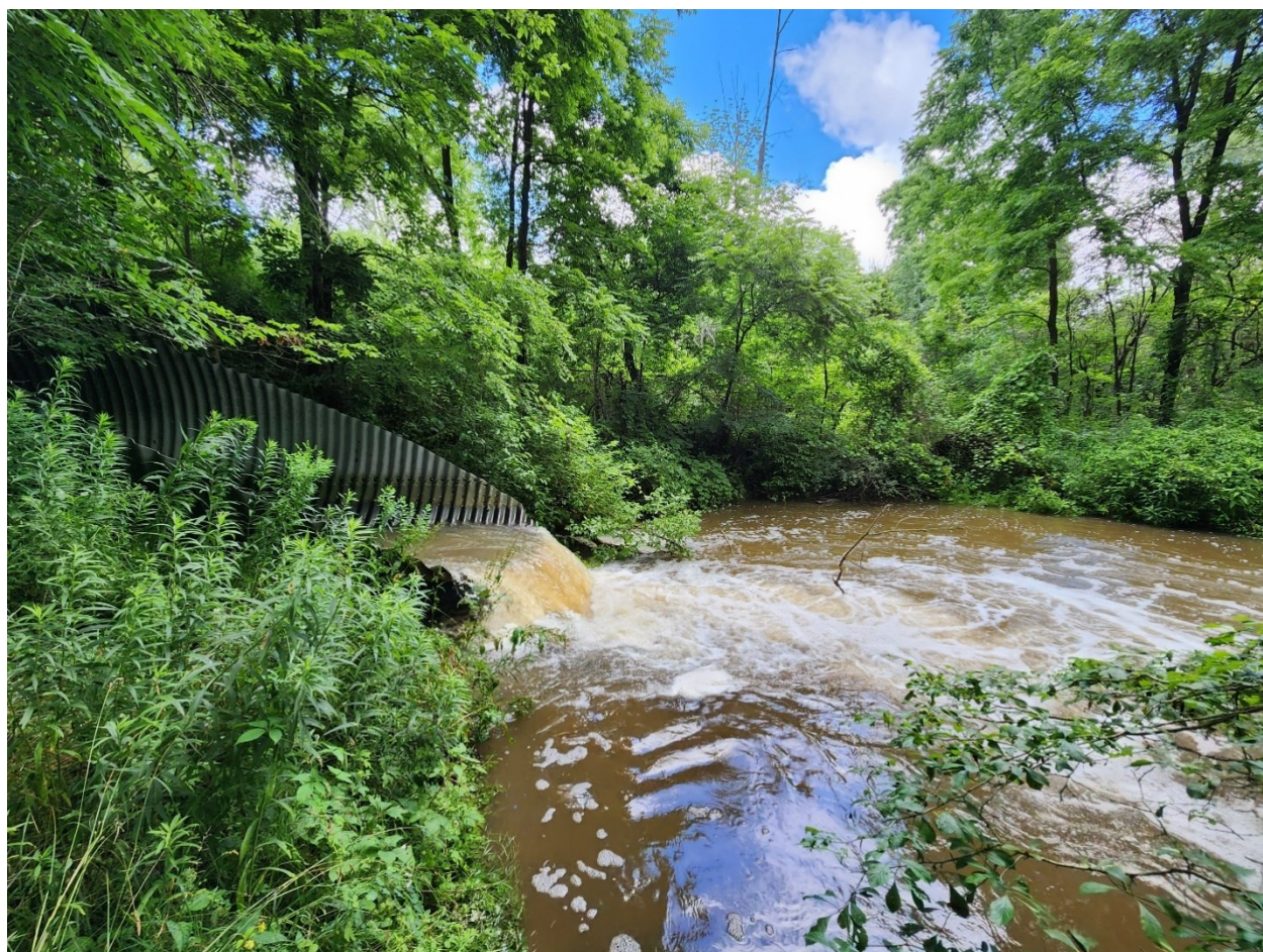
Figure 1. ON_LE_002: Burgess Creek Perched Culvert where the recommended restoration action is to replace the perched culvert and improve physical in-water features for native species.
