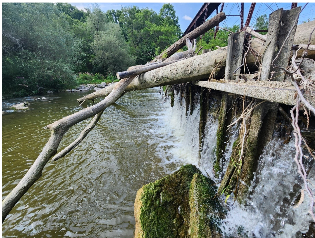
Figure 2. ON_LE_039: Black Bridge Rail Dam where the recommended restoration actions are to rebuild the barrier to block Sea Lamprey passage, protect downstream conservation area from erosion due to dam failure, and to construct a fishway that allows for passage of species other than Sea Lamprey or Rainbow Trout.
