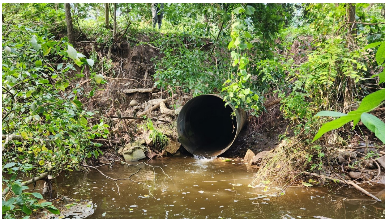
Figure 4. ON_LE_024: Charlie Creek Perched Culvert where the recommended restoration action is to remove the perched culvert and naturalize the stream.
