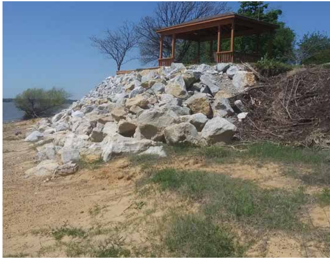
Figure 2. Rock blanket at Site 1; large (beige) rocks placed in 2020; smaller (grey) rocks added in 2024.
